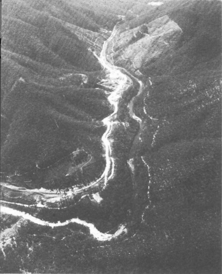
The Dartmouth Dam site, viewed from downstream, showing the Mitta Mitta River and the access road.
