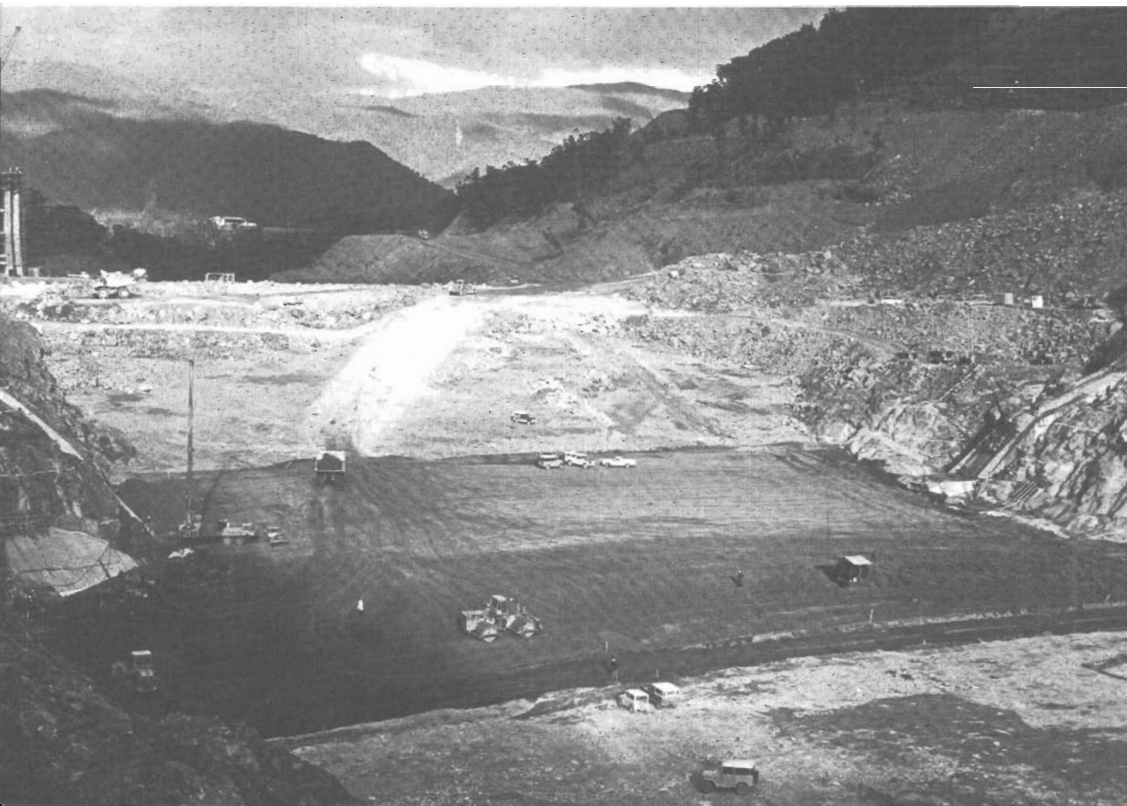
Embankment construction at the Dartmouth Dam site. The core zone in the centre is flanked by filter and rock zones.
